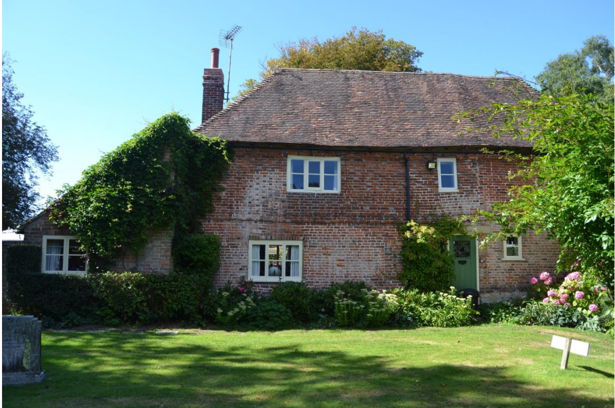
Figure 8: Farmhouse in the east of the borough - hipped roof with clay tiles; red brick and timber casement windows, typical of this area.
